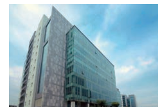
ABS Aircon Engineers Private Ltd. (India)
