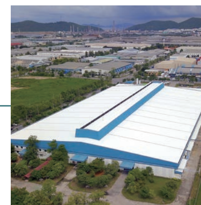
Fujitsu General (Thailand) Co., Ltd. (Thailand) Factory-2
