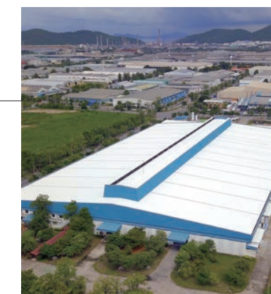
Fujitsu General (Thailand) Co., Ltd. (Thailand) Factory-2
