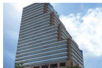
Fujitsu General (Thailand) Co.,Ltd. Bangkok Office (Thailand)
